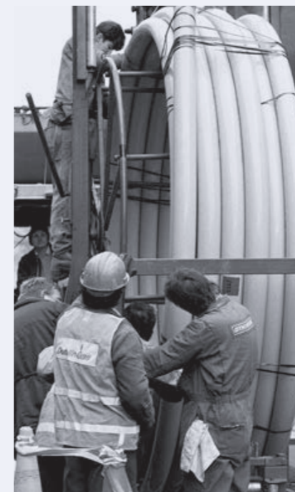
Dublin Gas Construction 1990
